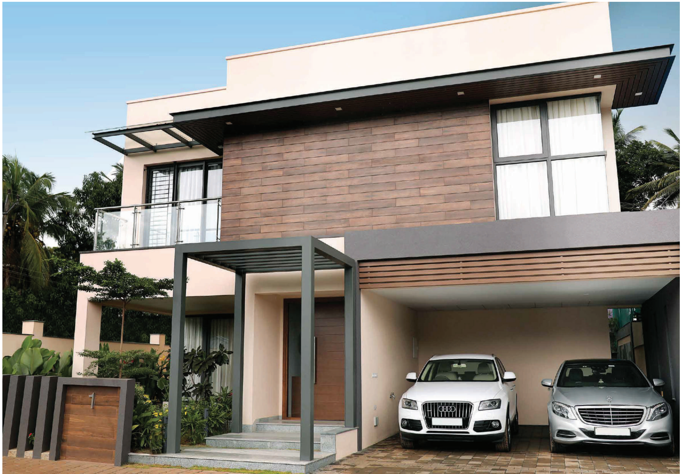
Type 1 Villa Elevation - Actual photograph shot at site
